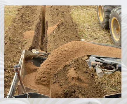
An envelope material is used to improve the permeability of the drain excavation and and soil surrounding the drain pipe, to prevent soil material from entering the pipe, and to protect the pipe under difficult installation conditions
